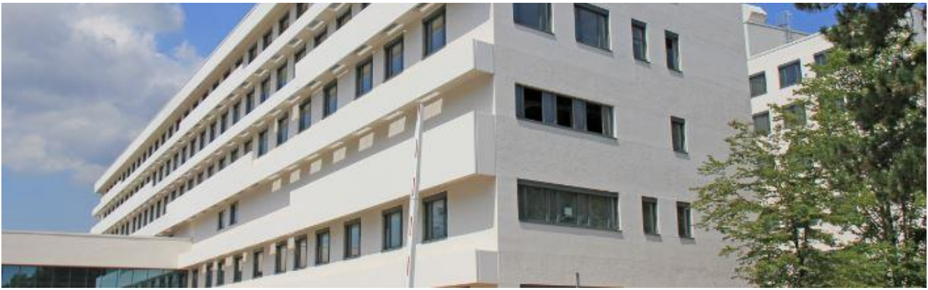
The new hospital building provides more than 660 beds for patients and another 40 beds in an outpatient clinic in addition to eleven operating theatres. Over 1600 employees will be working in the new building. © Klinikum Frankfurt Höchst
